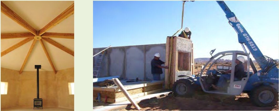
Figure 14. Left: Interior of a finished Elder Hogan home (Photo: Harry Connolly). Right: Construction of straw bale exterior walls (Photo: Nathaniel Corum). Photos used with permission from Sustainable Native Communities Collaborative.
