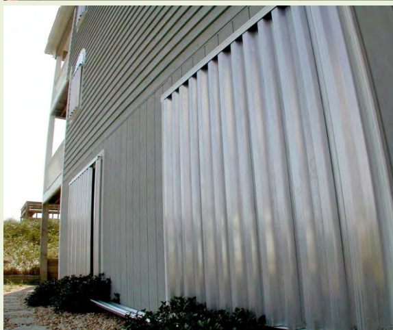
Figure 16. Top: Gable end wall failure occurs when walls lose support along the top edge; as a result, sheathing is blown off, causing the walls to fall inward or outward (South Carolina Department of Insurance). Middle: Integral gutters on a roof will not be torn away from the structure during a high-wind event (FEMA). Bottom: Storm shutters installed over doors and windows on a residence (Photo by Dave Gatley / FEMA).
