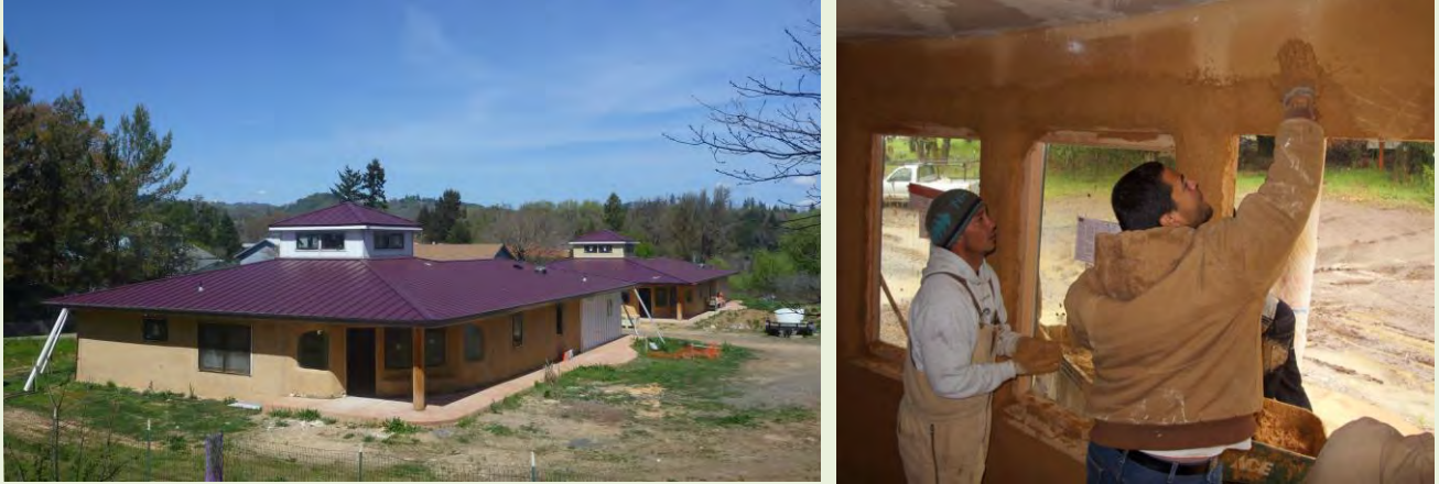
Figure 15. Left: Homes constructed for the Pinoleville Pomo Nation Homes project. Right: Applying earth plaster on an interior wall. Photos used with permission from Sustainable Native Communities Collaborative.
