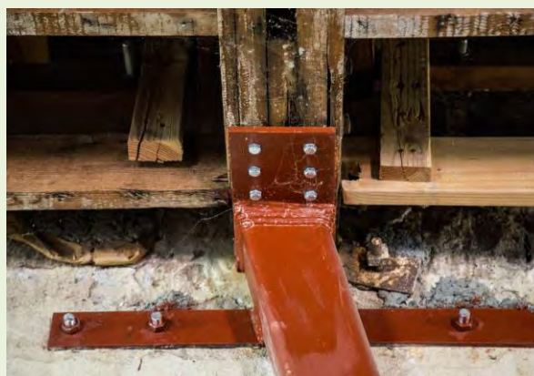
Figure 19. Photos of a secondary steel structural support inside the historic Borreo Building on Third Street in the city of Napa, California, which survived a magnitude 6.0 earthquake on August 24, 2014, with minor damage (Christopher Mardorf / FEMA).
