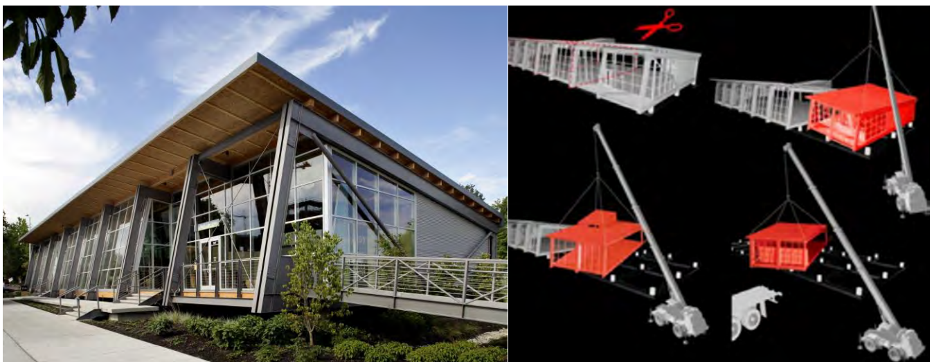
Figure 13. The South Lake Union Discovery Center in Seattle was designed for future transportation, reassembly, and reuse in a new location. The building separates at three integrated joints to break into four modules that can be moved on trucks by streets (not freeways). The building sits lightly on the land atop short concrete piers, allowing the grade and vegetation to run uninterrupted beneath. Gangway ramps with hinged joints can adapt to the topography of future locations (The Miller Hull Partnership).
